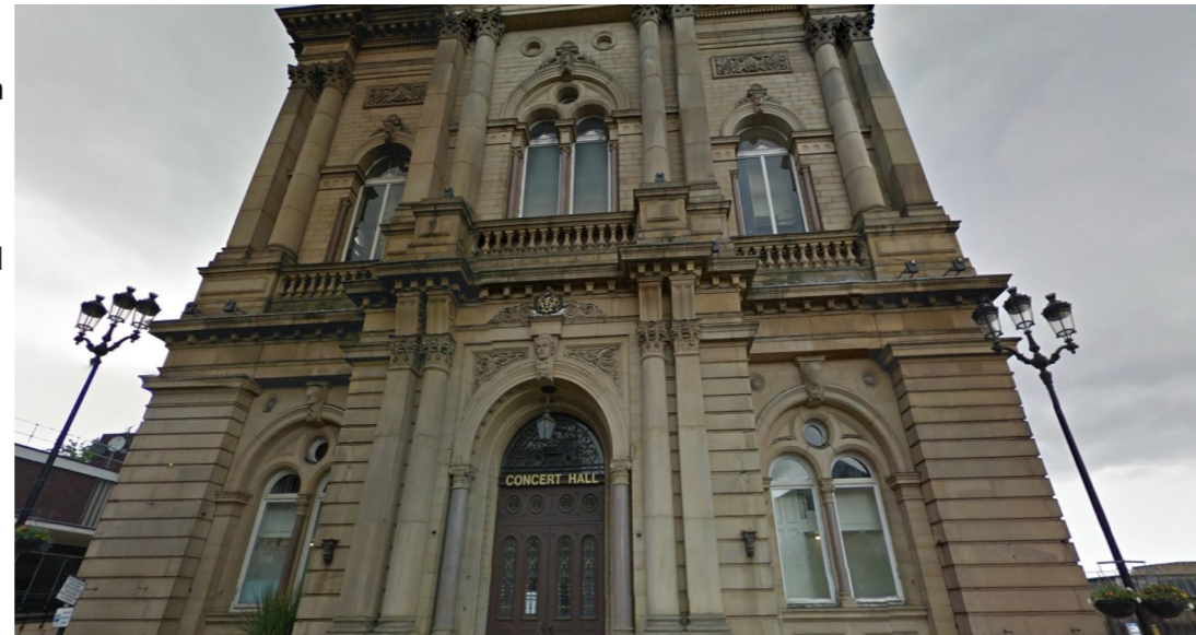
Above: Huddersfield Town Hall with gold standard heritage lighting unique to the town centre
