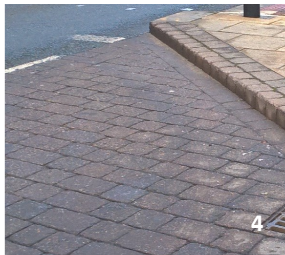
Above: (1) Asphalt roadways for streets with higher vehicular use have small unit paver or stone edge detail (2). Stone inset to inspection chamber also to be used (3) and (4) Small unit paver/setts could be used for laybys
